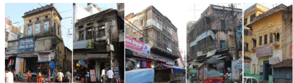
Fig. 11: Dilapidated old buildings Source:(Author)
